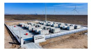
completed in just 19 days. The liquid-cooled energy storage containers are equipped with 314Ah batteries developed and produced by Narada's Base in Jiuquan. These batteries offer a cycle life of 12,000 times and a battery life of up to 20 years, while also providing a cell energy exceeding 1000Wh and a volumetric energy density exceeding 390Wh/L.
